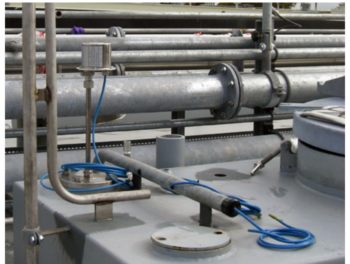
Fig. 3: Temposonics Level Plus® transmitter installation.
